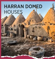
The conical domed house architecture in Harran was developed to protect against the extreme heat, which can reach 45 degrees Celsius in summer. These houses provide cool spaces in summer and warm spaces in winter. The ventilation opening left at the top of the domes allows light and air into the room, also serving as a chimney.
